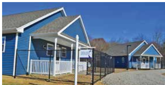
These two new canine cottages will make up the total of 8 canine cottages when the project is completed.
