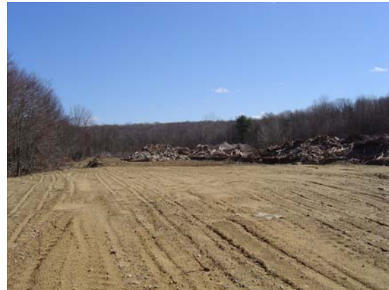
View of land in Ashford after demolition of existing buildings
