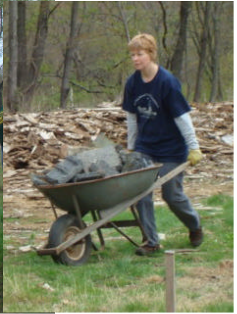
Kim Chagnon hauling concrete
